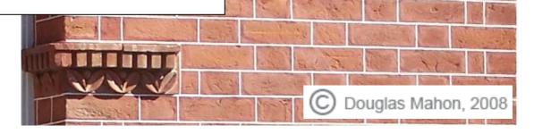
Our most popular method of pointing is RIBBON or HALFTUCK, a similar technique to TUCK although not as labour intensive and subsequently a cheaper option.
